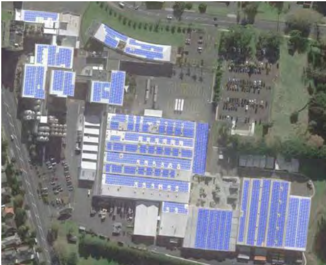
Figure 23: Rooftop Solar PV
